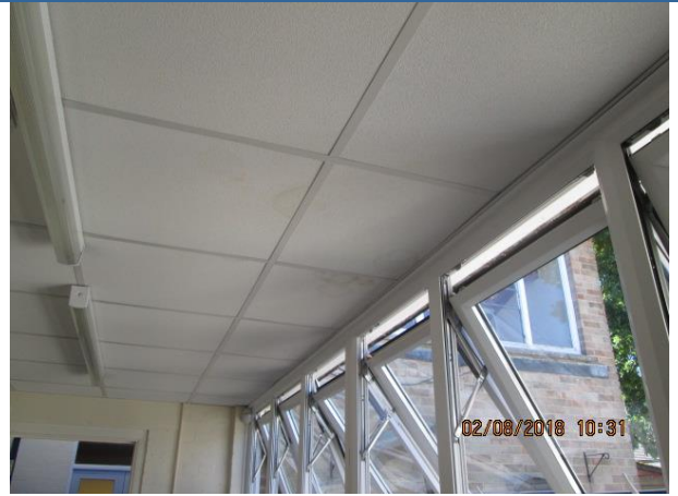
Ceiling tiles in grid below woodwool deck
