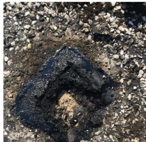
Core sample of Asphalt roof
