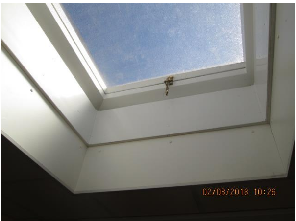
Internal of rooflight
