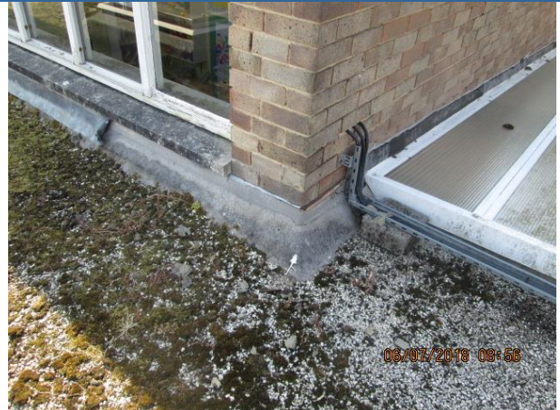
Main roof flashing example – pitched roof 5
