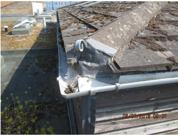
Patch repair to hall roof hip tiles
