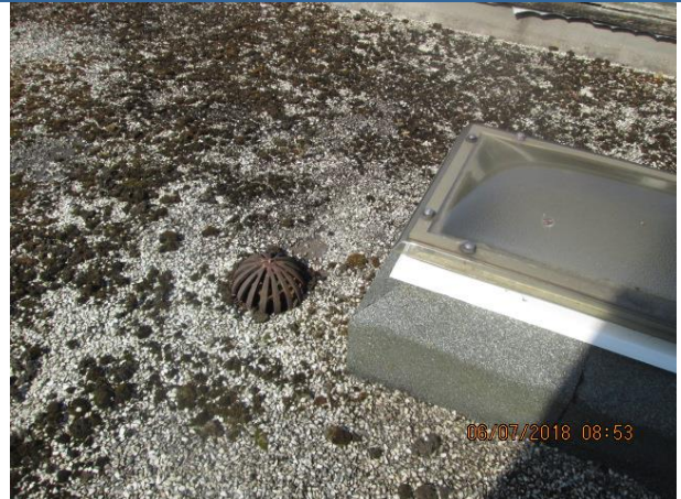
Main roof gully outlet and rooflight
