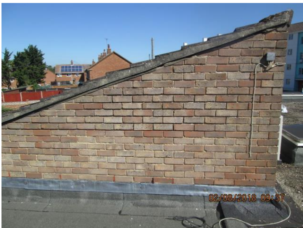
Pitched roof 2 – gable end South
