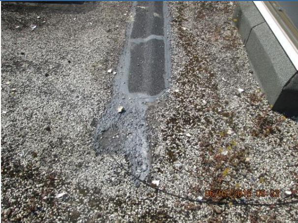
Main roof - patch repair
