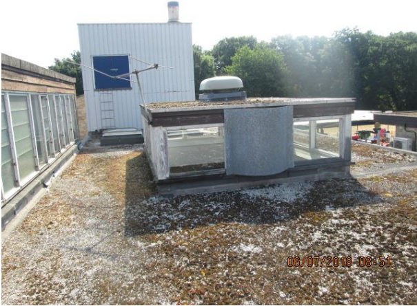
Main roof, raised kitchen roof and tank room in distance
