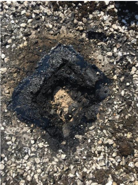
Core Analysis sample showed the deck to be dry.
