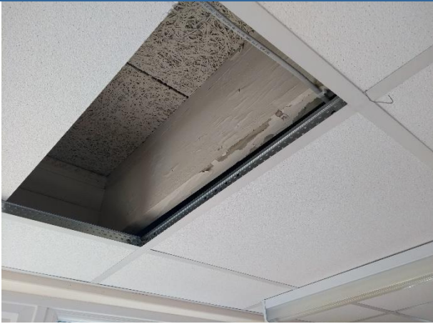
Woodwool deck below asphalt, timber joist and ceiling tile lifted out
