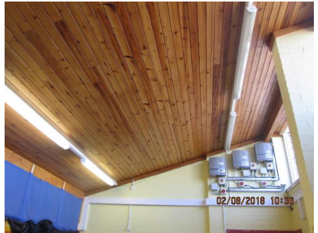
Interior of pitched roof 5 – no obvious movement
