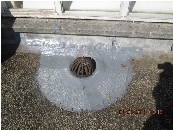
Recent Acrypol patch repair to asphalt roof adjacent to pitched roof 3
