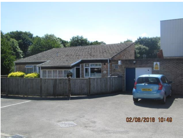
Caretaker's bungalow – North elevation
