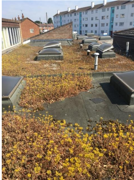
This picture shows an overview of the main roof.
