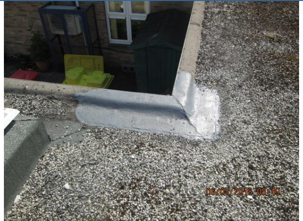
Main roof – edge patch repair
