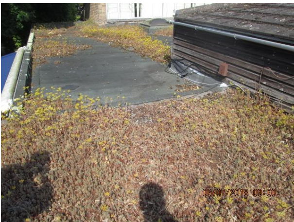
Small felt roof 2 in back ground, main roof in fore ground
