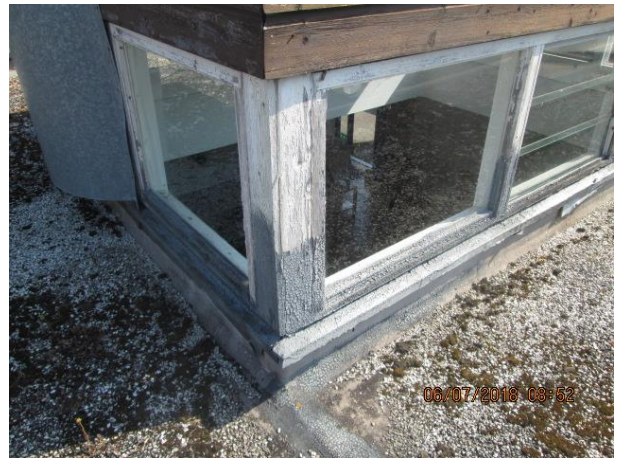
Clerestory kitchen windows
