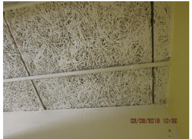
Underside of woodwool decking below asphalt roof
