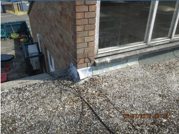
Main roof flashings and high level windows
