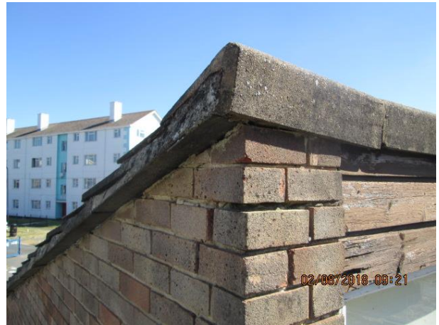
Pitched roof 1, lifting and opening mortar joints
