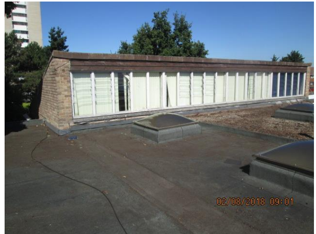
Felt roof 2 swept of debris and plant growth
