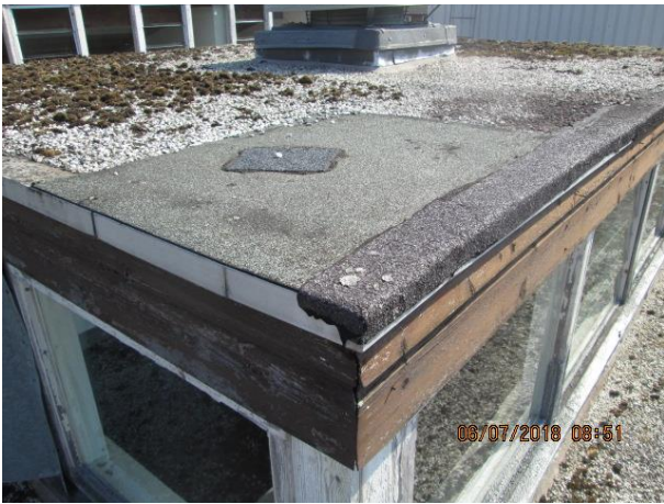
Kitchen roof – patch repair
