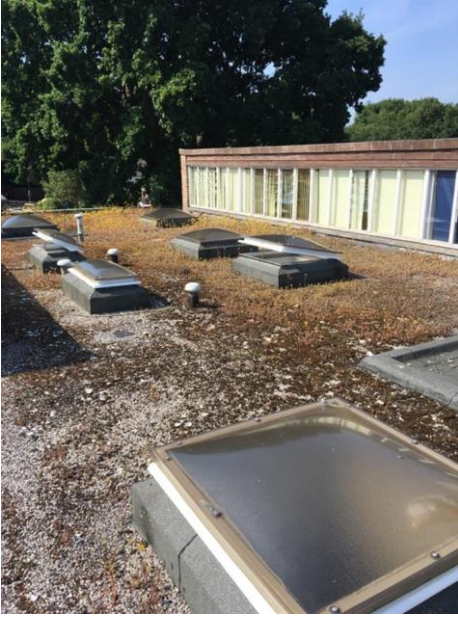
Alternative view of the main roof.
