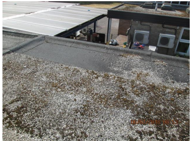
Patch repair to main asphalt roof adjacent small roof 3
