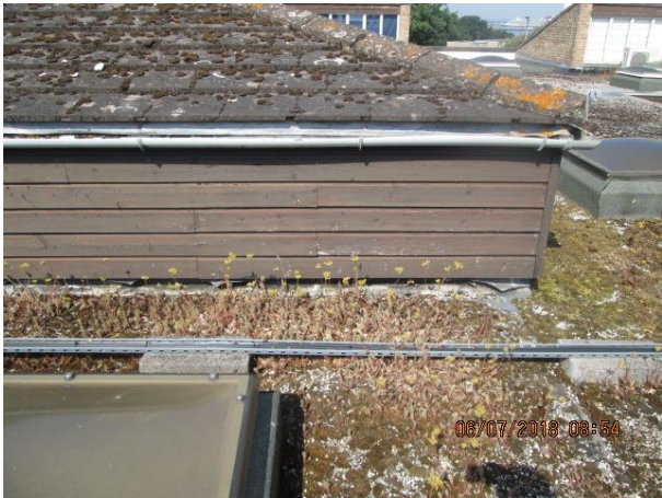
Hall roof above main asphalt roof Service trunking on blocks
