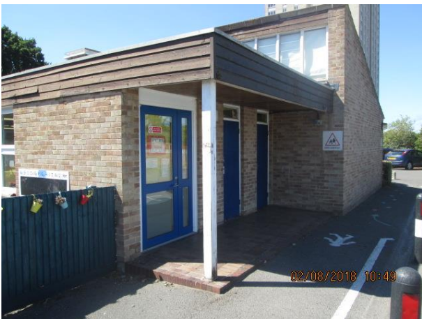
Corner post under asphalt roof
