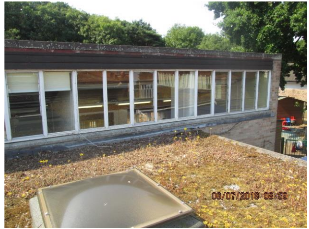
Main roof and high level glazing, pitched roof 4
