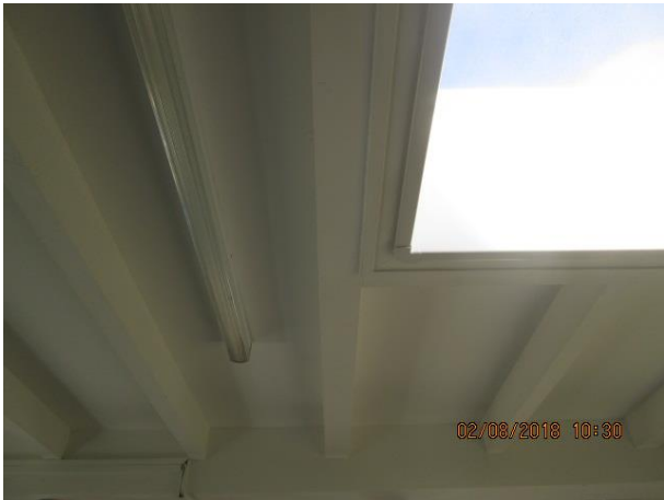
Fixed (probably plasterboard) and painted ceiling below felt roof 2
