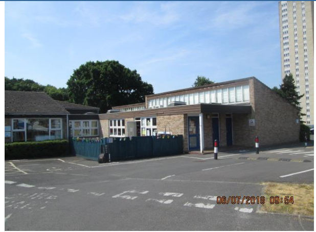
Front elevation of school
