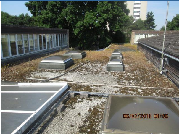
Main roof, pitched roof 4 on left, hall roof on right
