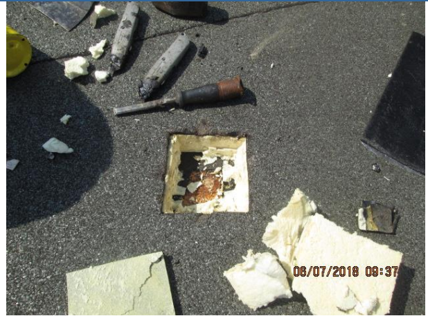
Core Sample of small felt roof 1
