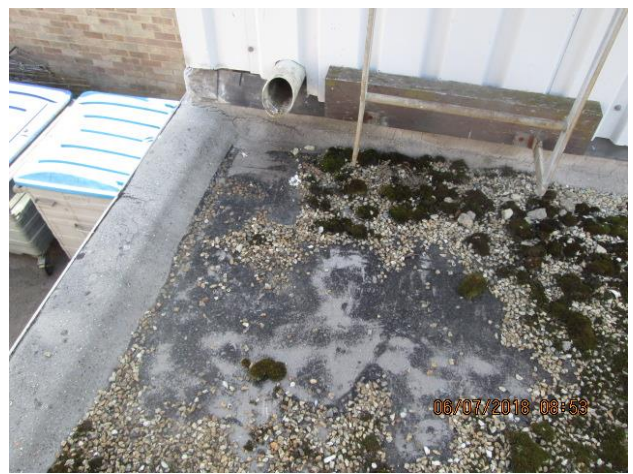
Gutter outlet of tank room roof onto main roof
