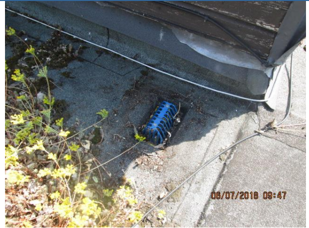
Small felt roof 2 – cleared gully
